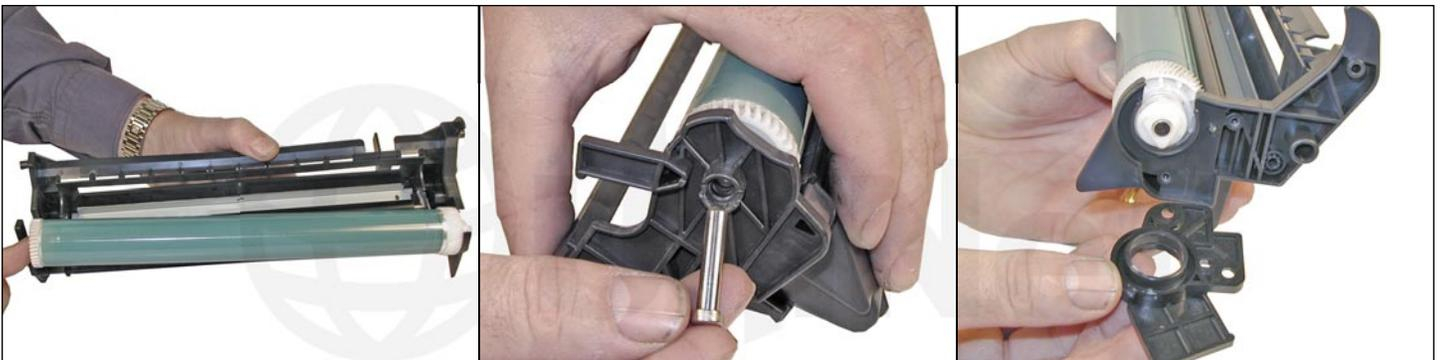
20. Coat the OPC drum with the Kynar, and replace the OPC drum, metal axle, and plastic drum bushing.
